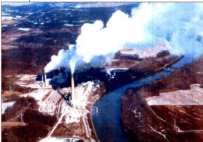
Coal-Fired Power Plant
