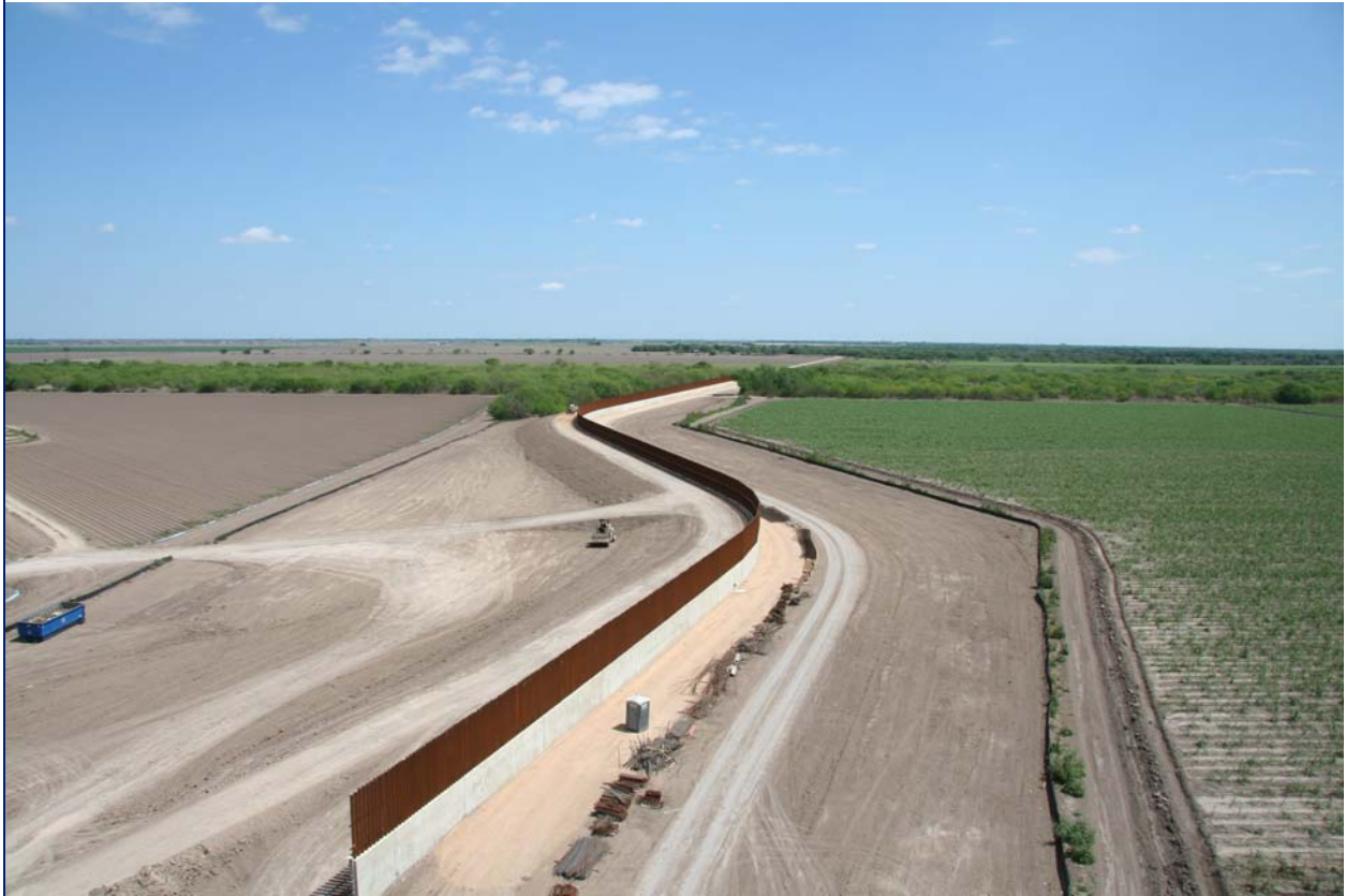
US Border Fence: Rio Grande Valley, Texas
