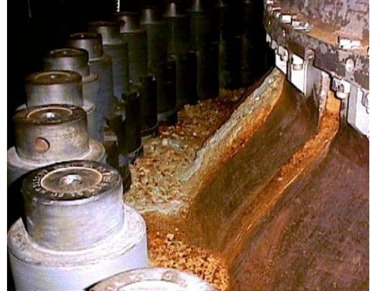
Pictures taken in 12RFO of the reactor vessel head flange showing boric acid with rust flowing out of the weep holes.
