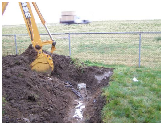
Excavated underground pipe
