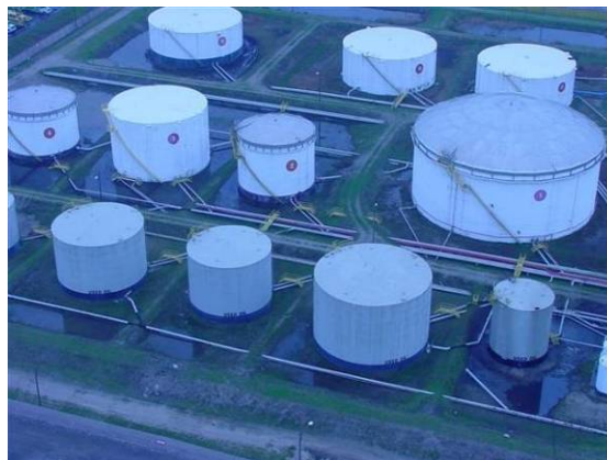
Aerial view of tank farm
