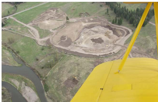
Discharge from pond to river
