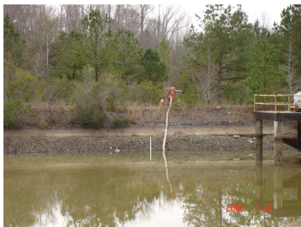
Pumping water from lagoon into creek
