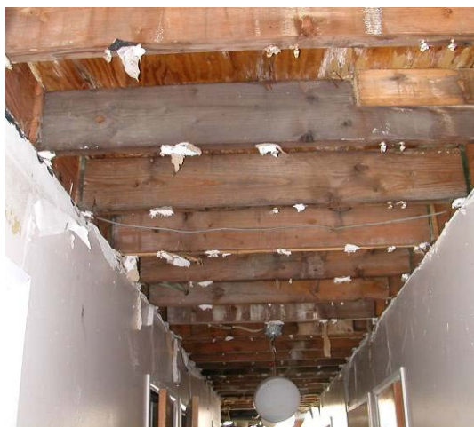
Apartment ceiling after illegal asbestos removal
