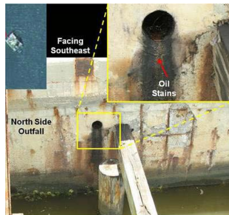
Oiled outfall at Bayou St. Denis facility
