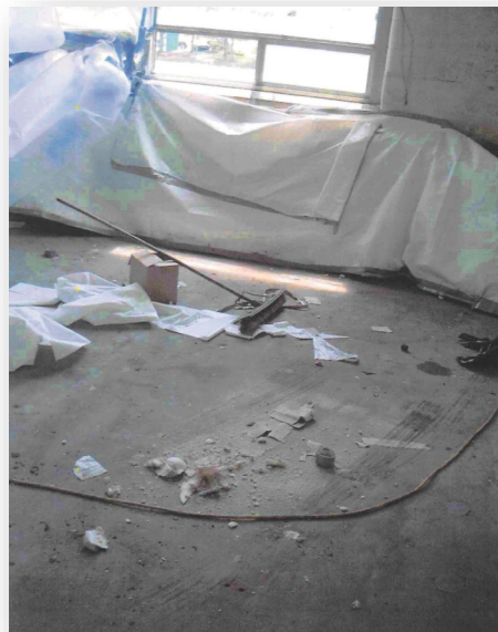
Loose, dry asbestos, and breached critical barriers.
