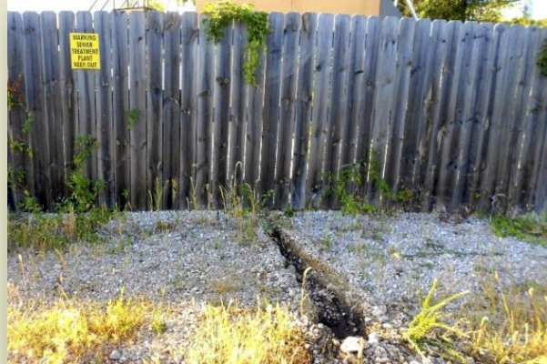
Trench dug to allow sewage to flow from facility
