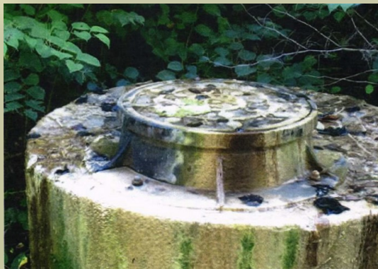
Manhole cover stained with leachate
