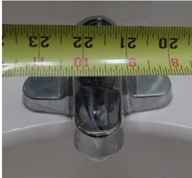
Dimension from side wall to centerline of lavatory in Unit 3-104 hall bathroom.
