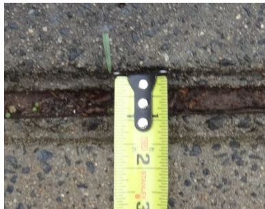
Measurement of gap width.
