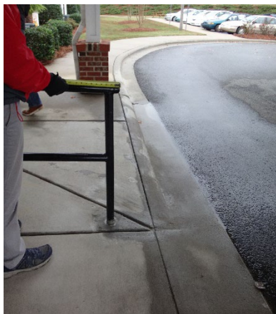
Handrail at ramp leading to building entrance.
