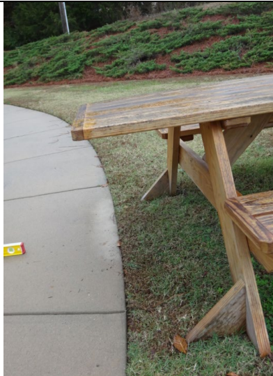
Close up of west end seating space overhanging sidewalk.
