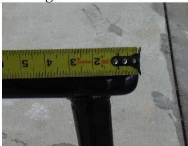
Handrail at ramp leading to building entrance.
