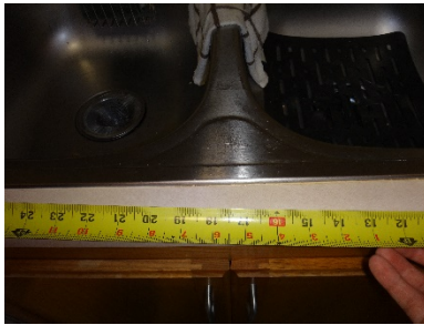
Sink centerline, Unit 109.
