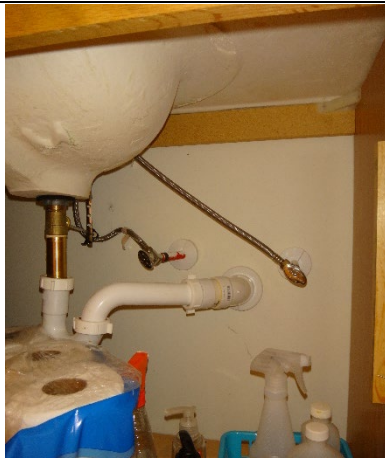
Base cabinet interior of lavatory in Unit 214.
