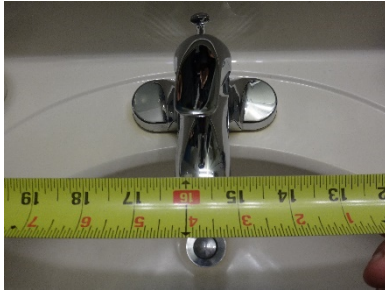
Measurement to centerline of hall bathroom lavatory in Unit 2005.
