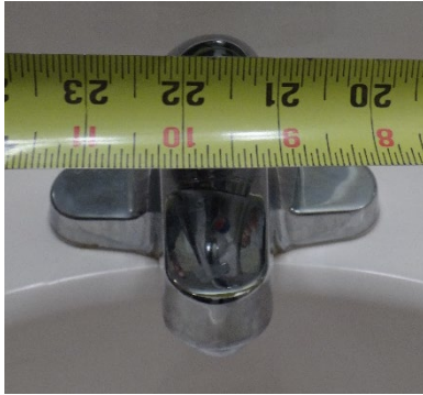
Dimension from side wall to centerline of lavatory in Unit 3-104 hall bathroom.
