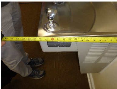
Projection from the wall.
