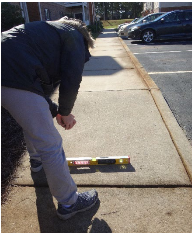
Curb ramp at the east entry of Building 3.
