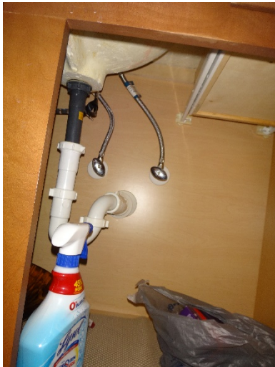
Interior of vanity in Unit 3-104 hall bathroom.
