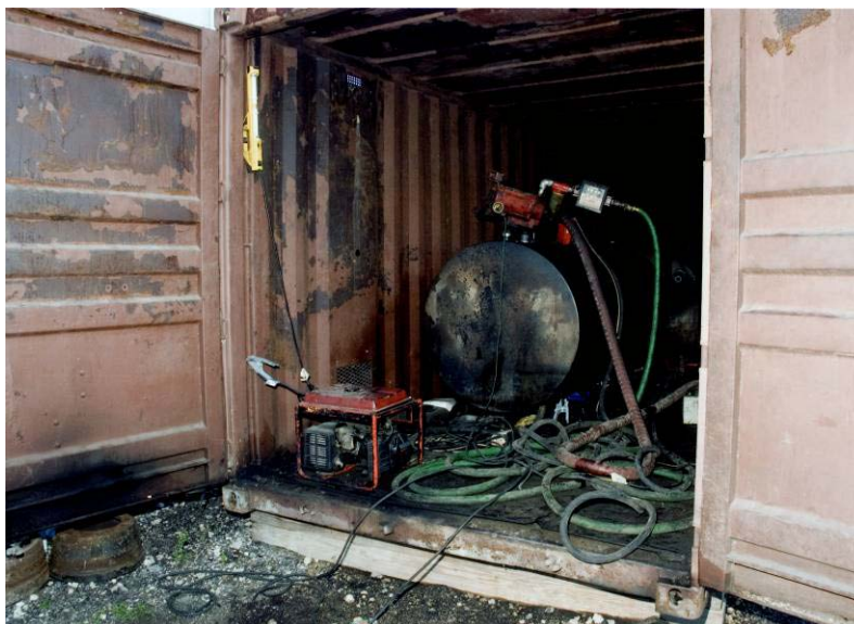
Container with concealed storage tanks
