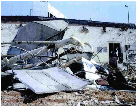
Asbestos-covered demo debris
