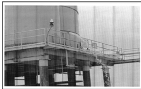
Illegal discharge of water into Breton Sound
