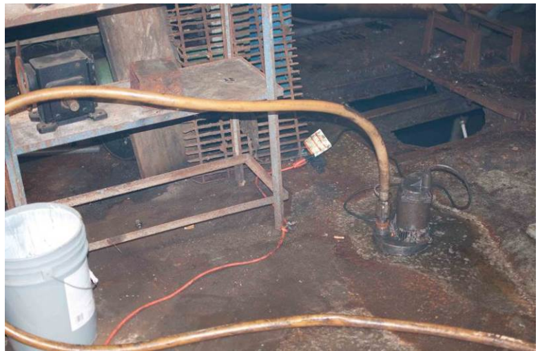
Pump used to bypass pretreatment system
