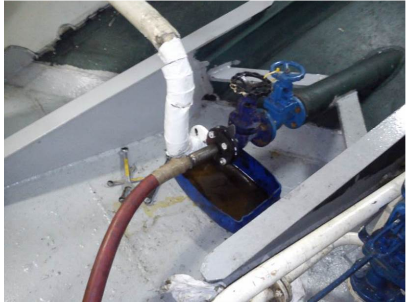
Bypass discharging through seawater supply line
