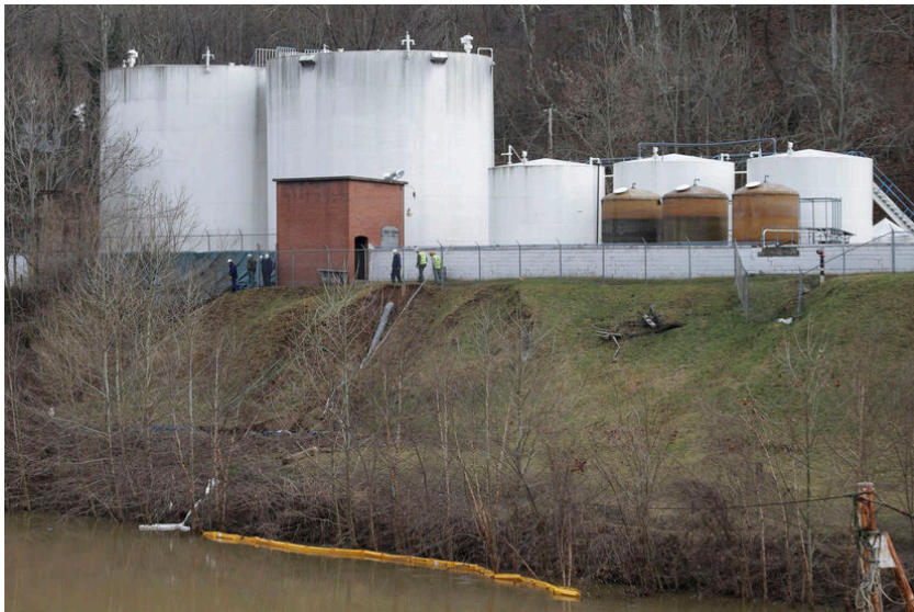
Site where chemical was spilled into river
