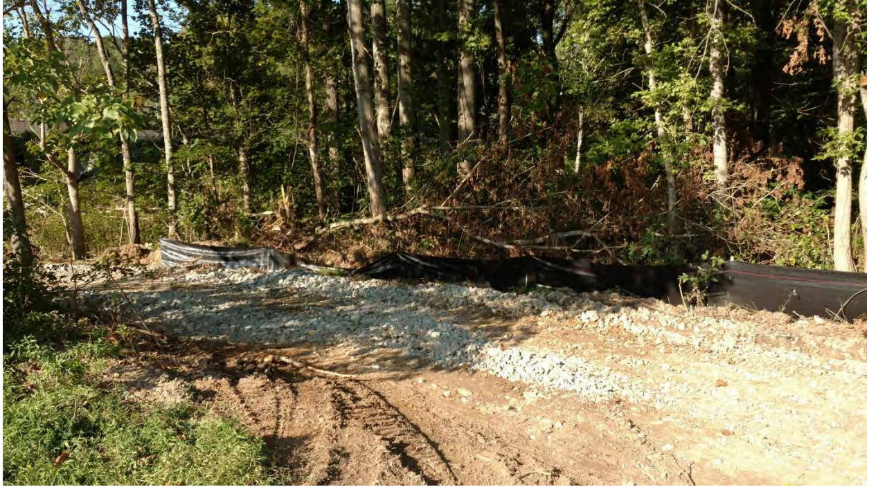
9. Access road down to floodplain causeway with silt fencing in place, view north (9/7/16)
