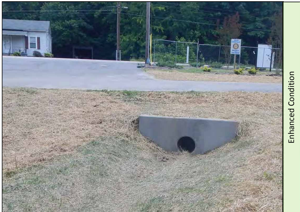
Picture 8: New headwall added to existing culvert.
