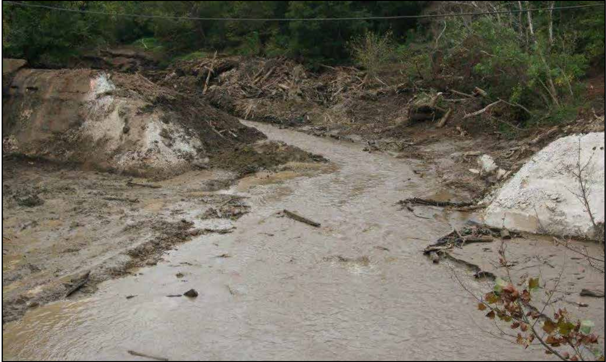
23. Sixty-five foot width base flow channel completed through Power Dam (9/22/16) (credit FORVA)
