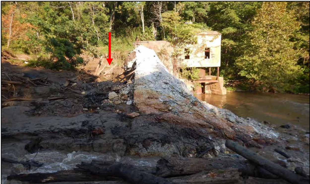
14. Exposure of existing scour hole (red arrow) above Power Dam, potentially leading to wetland headcut (9/7/16)
