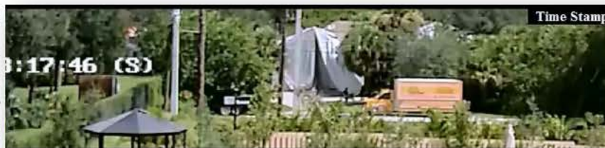
House prepared for fumigation
