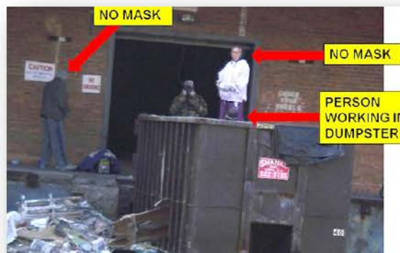
Workers clearing asbestos from dumpster
