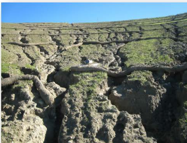
Slope erosion causing sediment to flow into pond
