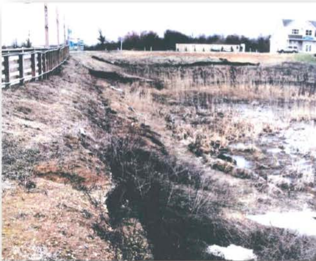
Road (top left) constructed through wetlands
