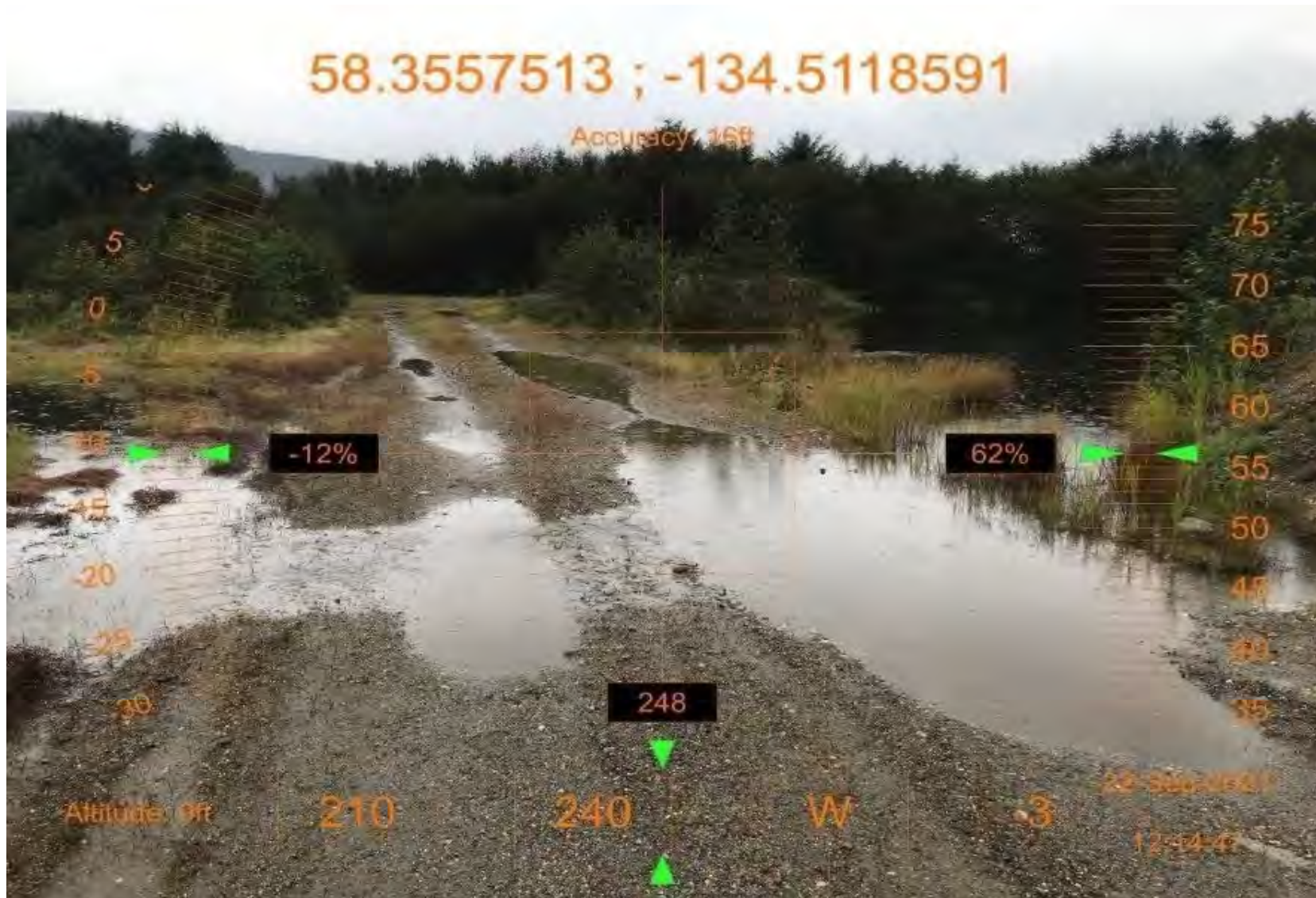
Photograph 17. View of the Connection Between S&S Pond 2 (to the left) and Pond 3 (to the right). View is to the southwest and water flows cross the road from right to left in the photograph.
