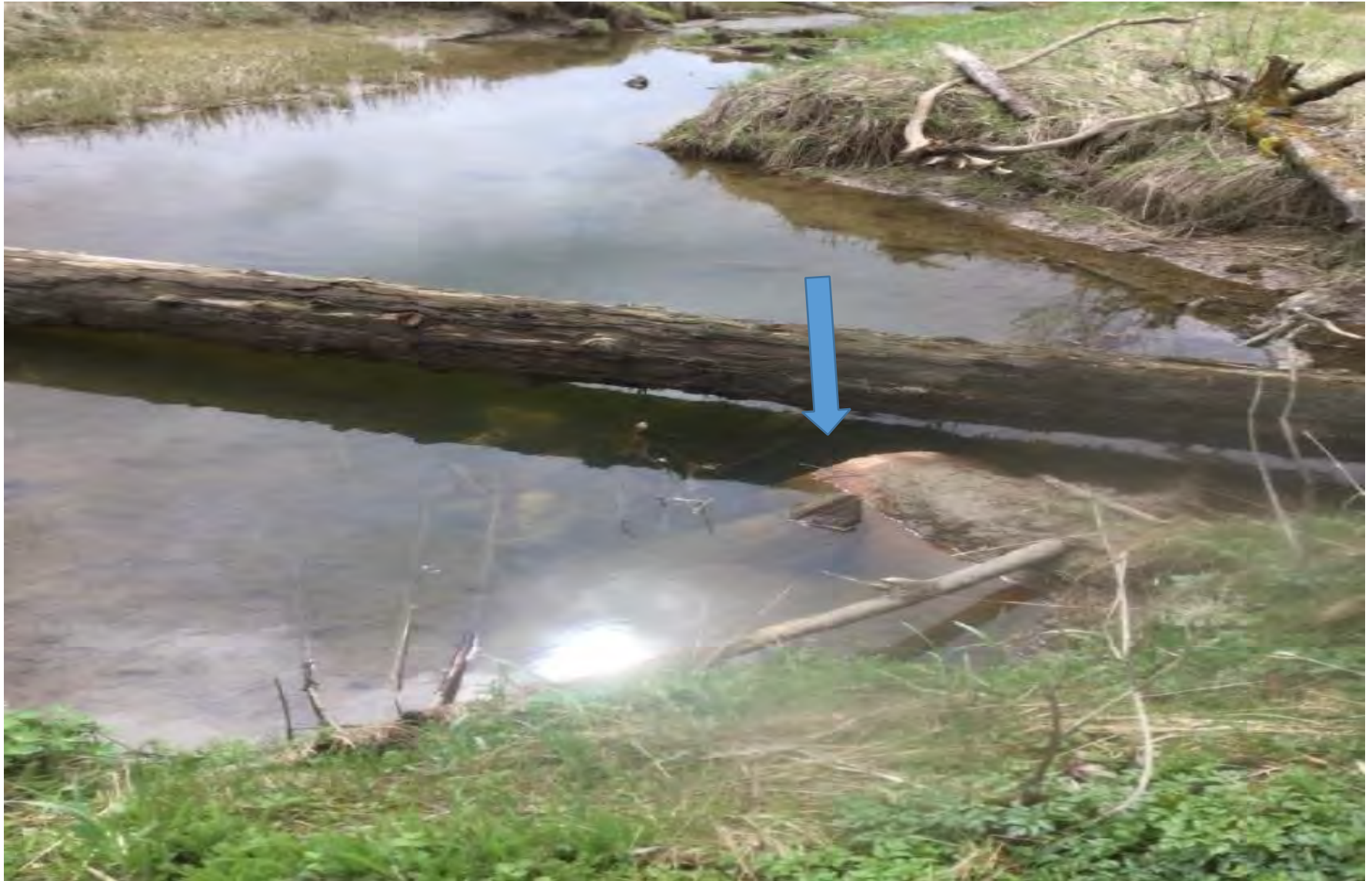
Photograph 18. The Downstream End of the Culvert (Blue Arrow) Connecting the South End of S&S Pond 1 to Lemon Creek.
