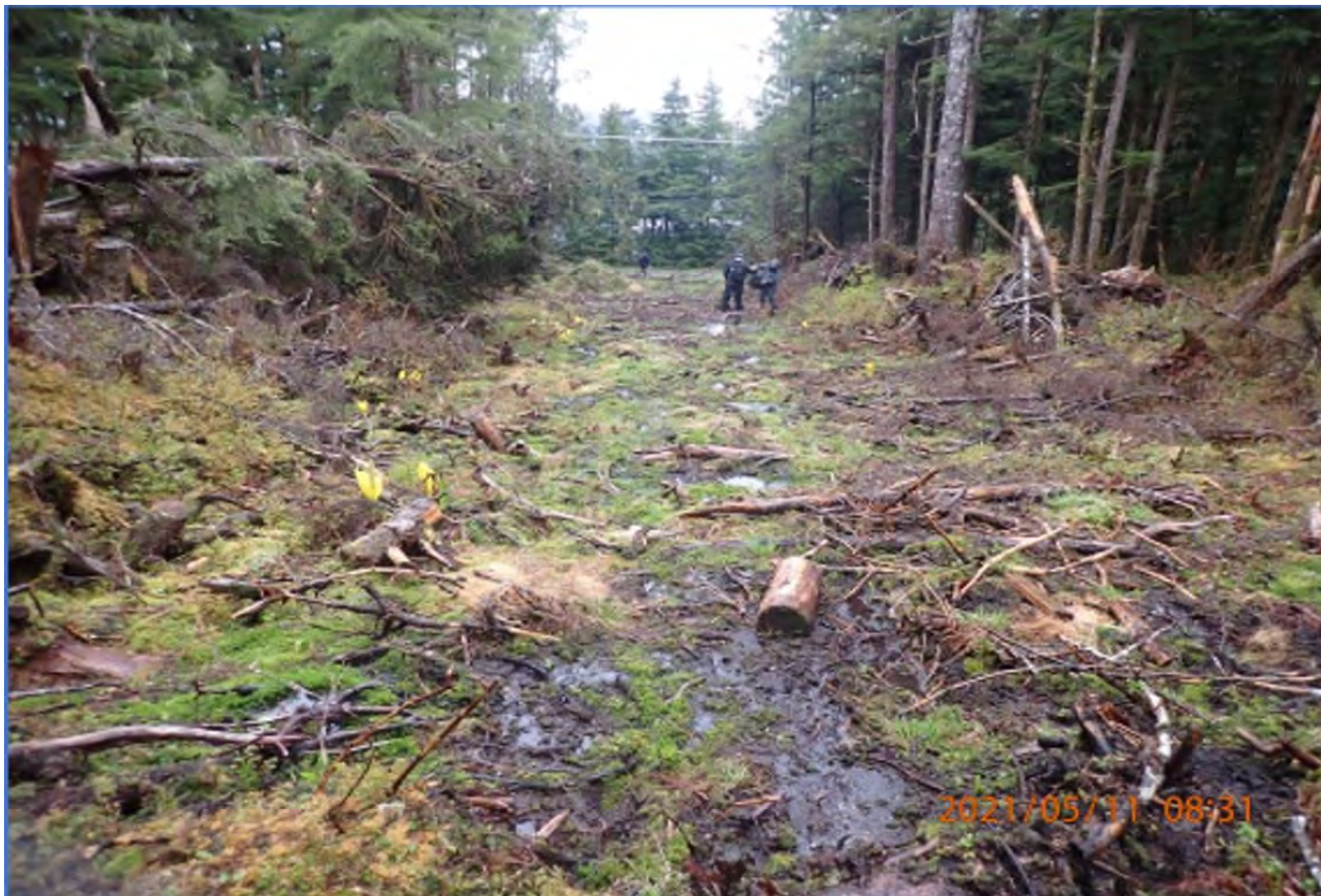
Photograph 1. Mechanically Cleared Forested Wetlands Along the Route of the “Pioneer Access Road” at Vista del Mar. View is downhill and to the south, towards Auke Bay.
