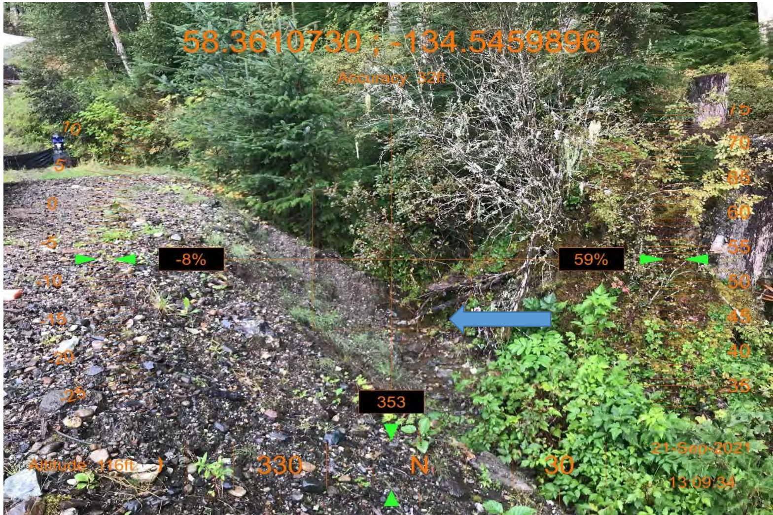
Photograph 12. Vista del Sol - Eastern Tributary Channel Filling and Lateral Confinement from Construction of a Housing Foundation Platform
