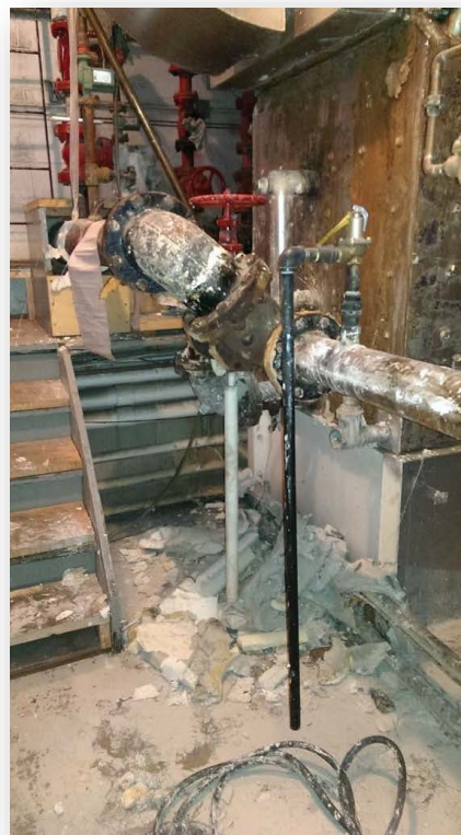
Asbestos waste in boiler room
