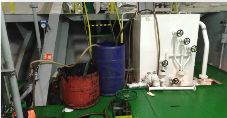
Illegal bypass hookup in M/T Zao Galaxy engine room
