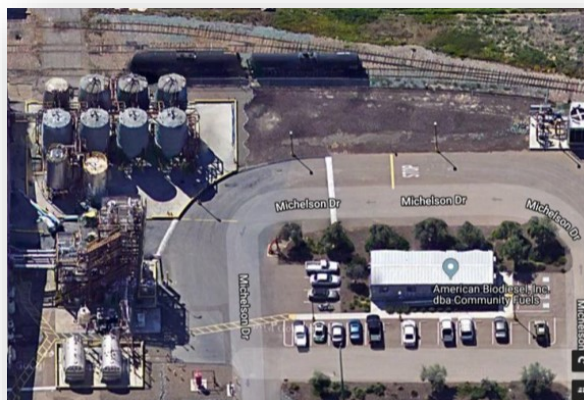
American Biodiesel facility
