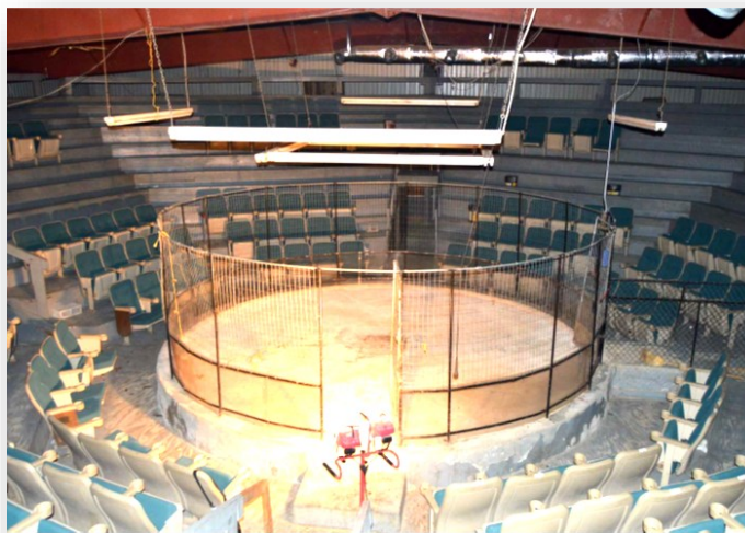
Arena prior to demolition
