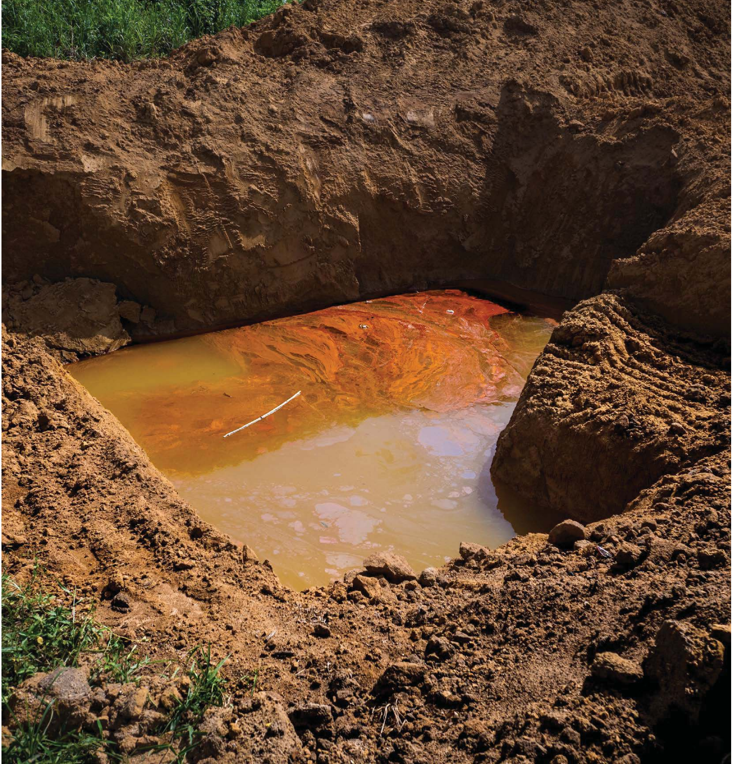
Lot 10: The excavated trench, with patches of oil and oxidized iron on groundwater. © Isaac Harry/cmapping.net Date: April 2020
