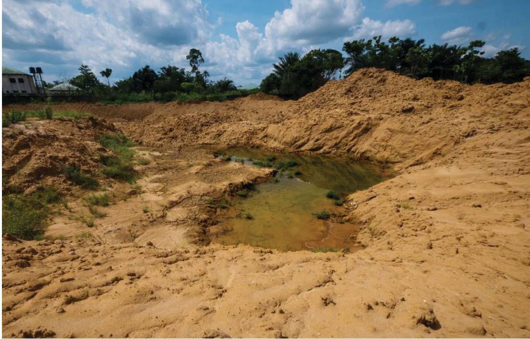
Lot 19: Untreated contaminated soil excavated in December 2019 is still in the open and placed side by side with treated soil. Since the excavated area isn't secured or properly separated, contaminated soil is washing into the treated soils around the area and those that have been backfilled in the trenches when it rains. © Isaac Harry/cmapping.net Date: April 2020
