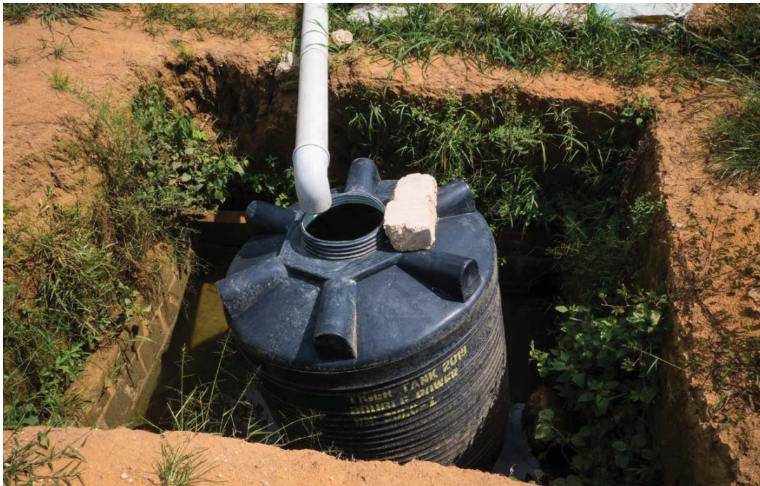
Lot 20: Poorly constructed sump. The sump isn't covered so when it rains the sump fills up and spills into the surrounding environment. © Isaac Harry/cmapping.net Date: April 2020
