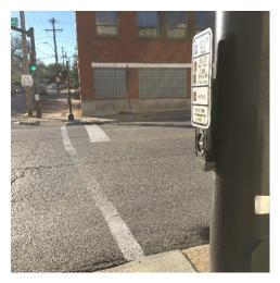
The audible and tactile "WALK" indication is the most critical information provided by an APS. *Id.* ¶¶28-29. When the visual pedestrian signal changes to the "WALK" signal, an APS emits a rapidly repeating percussive tone (between 8 and 10 ticks per second), which is much faster than and easily distinguished from the locator tone emitted during the "DON'T WALK" interval.
