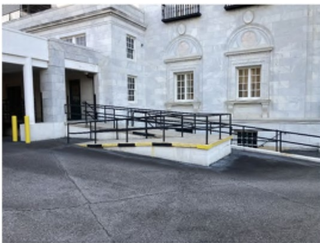
Augusta, GA – Prisoner delivery area without enclosed vehicle sallyport. A current Capital Security Program project including a sallyport is underway.
