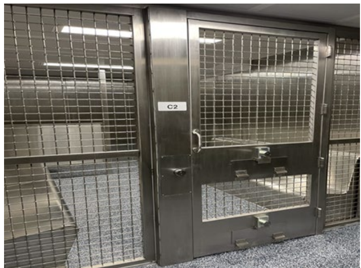
Marquette, MI – Renovation completed June 2021.
