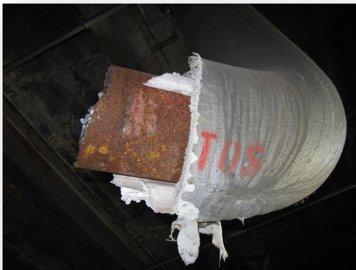
Asbestos-wrapped pipe
