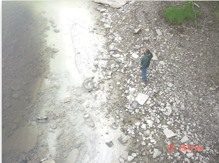
Concrete slurry visible in river
