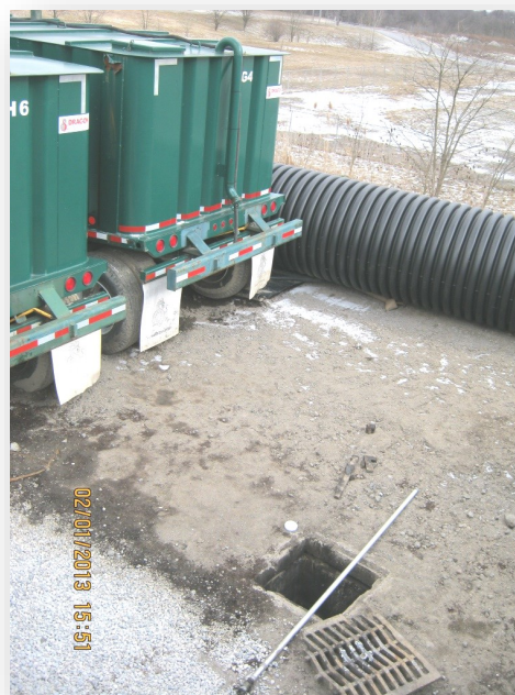
Stormwater drain used for illegal discharges
