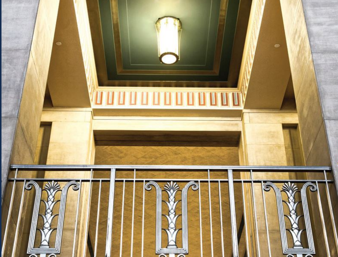
RFF building: Detail of aluminum railing along the stairway to The Great Hall
