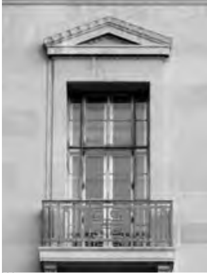
Detail of a fifth story window on the building's Constitution Avenue side.
