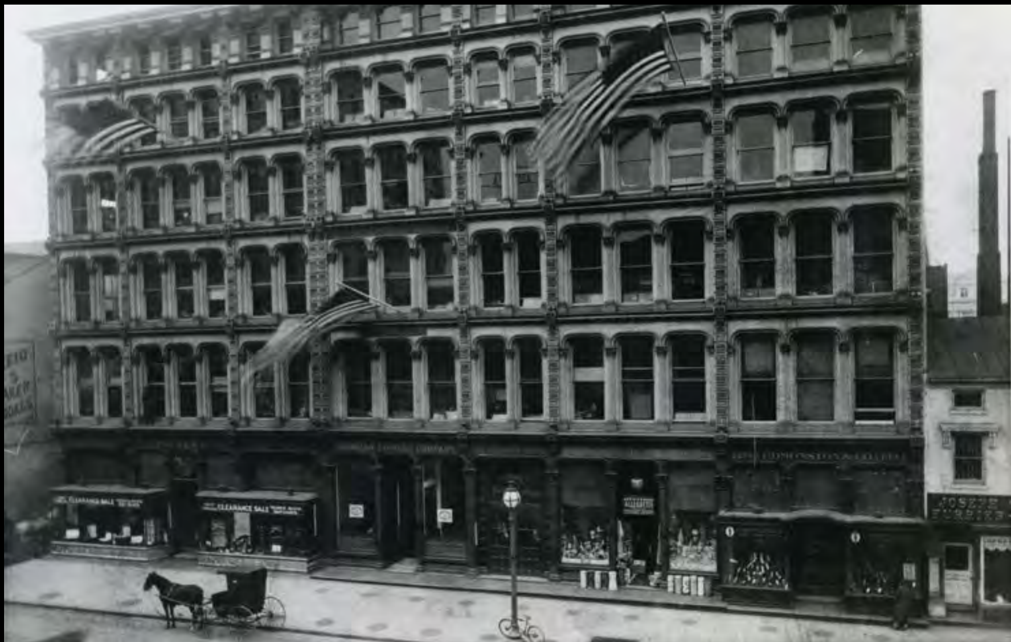
The Hooe Iron Building on F Street housed the Solicitor General and one of the Assistant Attorneys General and his staff. When it was built in 1873, it was Washington's largest cast iron front structure. The building was razed in 1926. 13
