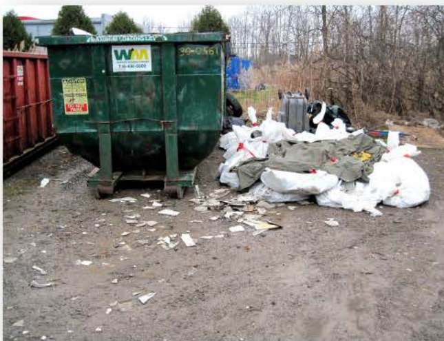
Asbestos-containing material left on ground outside Doctor's office
