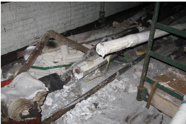
Asbestos insulation
