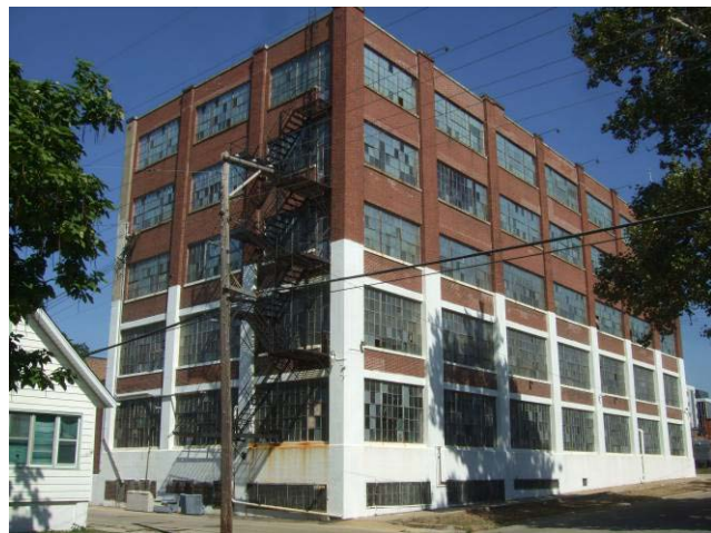
Building prior to demolition
