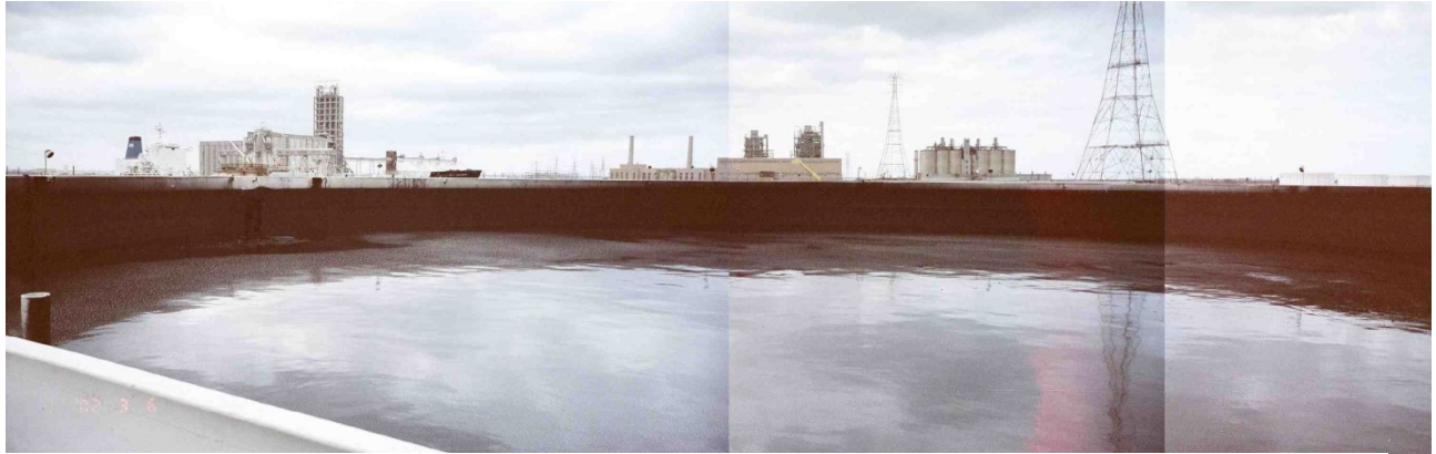
Tank with ten-foot-deep layer of oil
