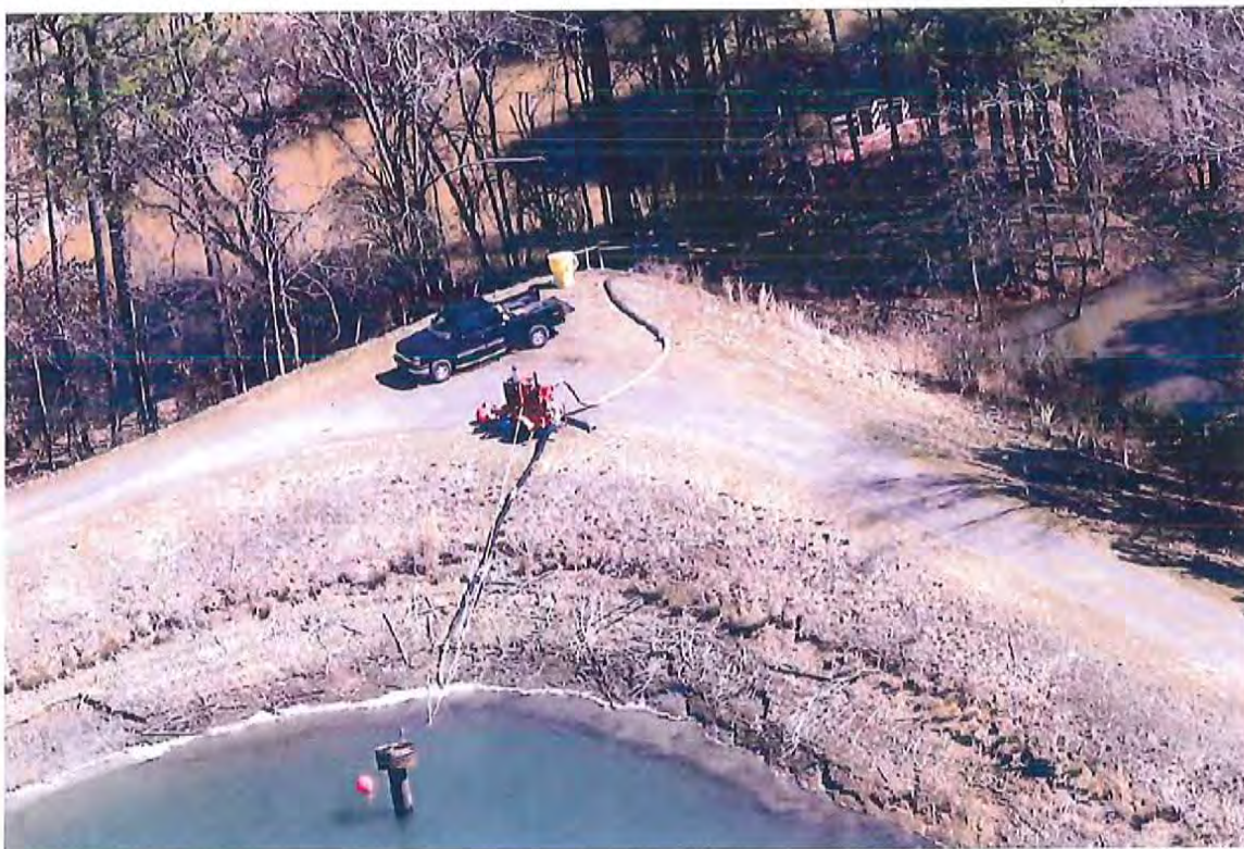
Photograph 8. 3/11/14 aerial photograph of CAPE FEAR 1978 coal ash basin with Godwin pump and truck.
