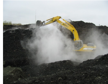
Workers battled recurrent fires at the Vinagro landfill (EPA)
